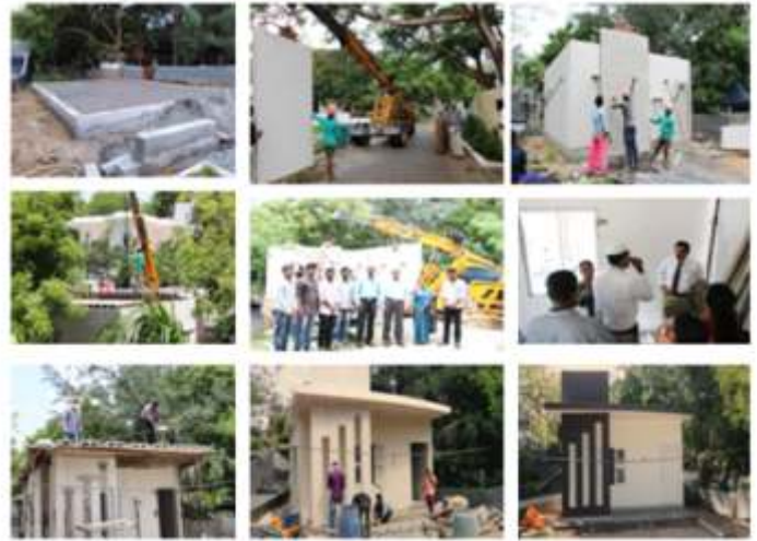
Construction of Affordable house using GFRG panels
