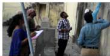
Condition Assessment of Crescent Matriculation H.S.School, Nungambakkam.
